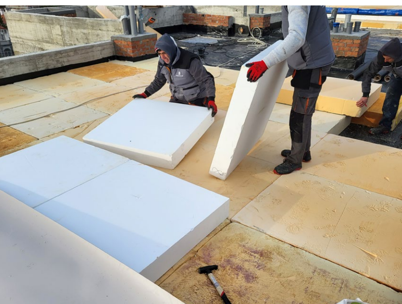
Postavljanje Austrotherm Resolution® i Austrotherm EPS® A150
