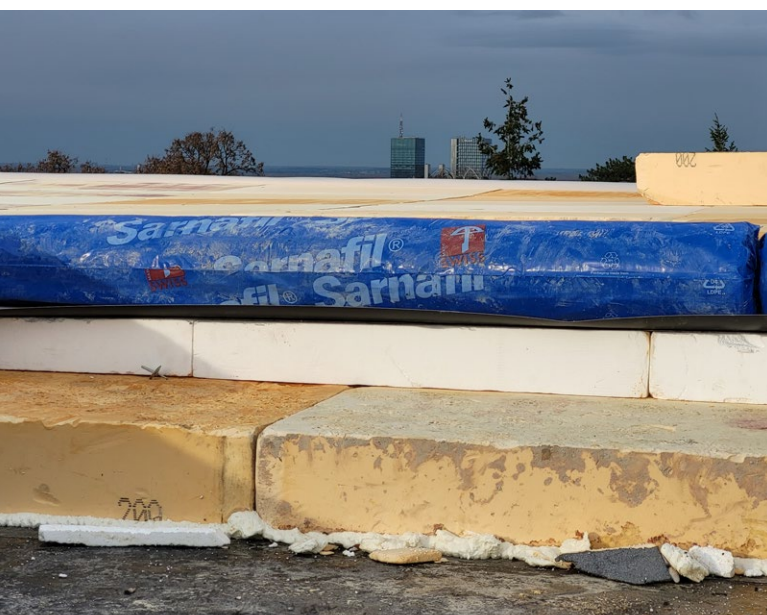
Postavljanje Austrotherm Resolution® i Austrotherm EPS® A150
