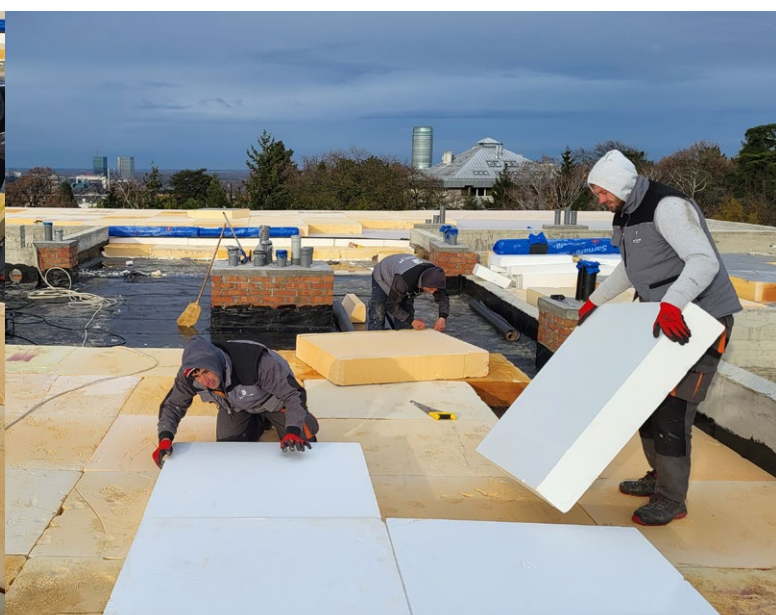
Postavljanje Austrotherm Resolution® i Austrotherm EPS® A150
